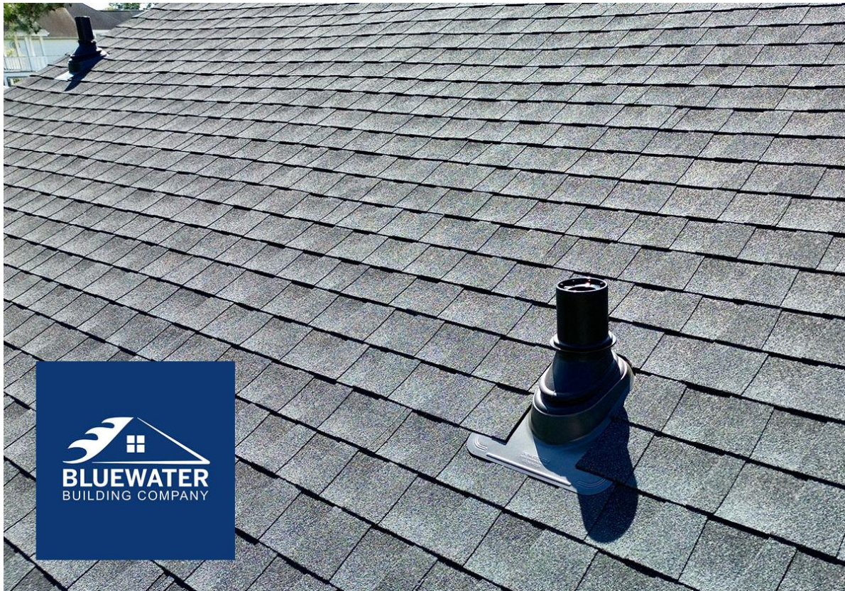
Bluewater Building Company installations of The Ultimate Pipe Flashing® with EASYSleeve®
