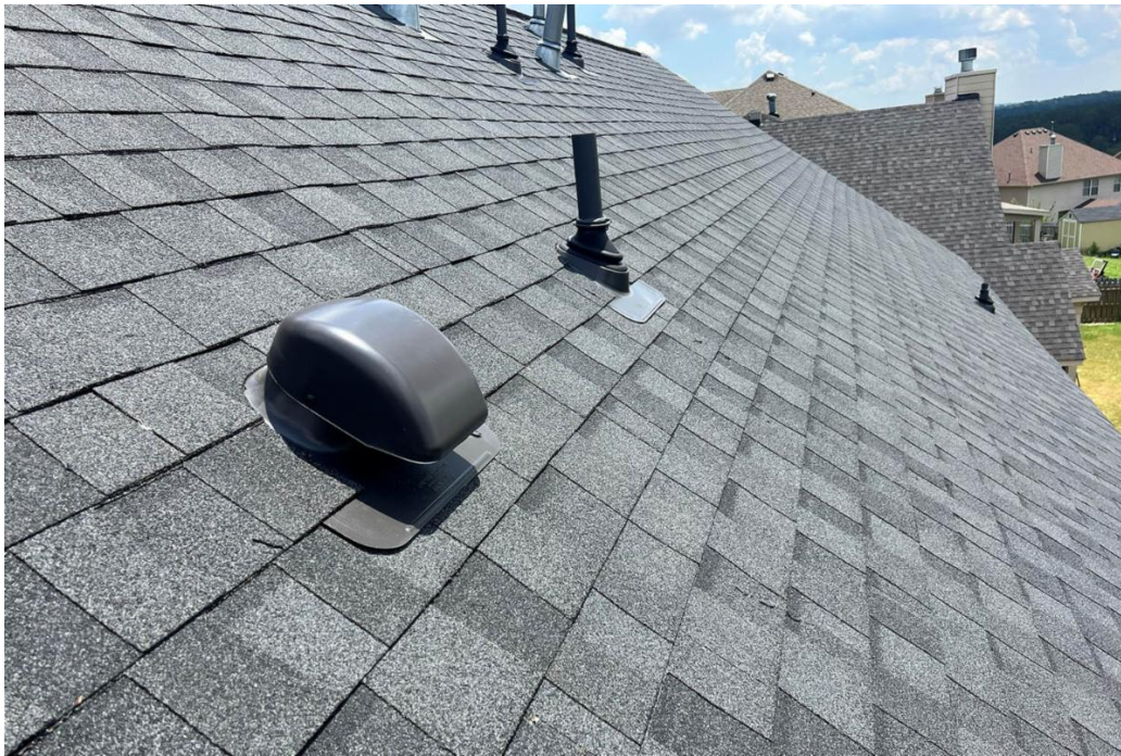
Crosby Roofing and Seamless Gutters installations of the Ultimate Pipe Flashing® and the Ultimate Bath/Dryer Vent
