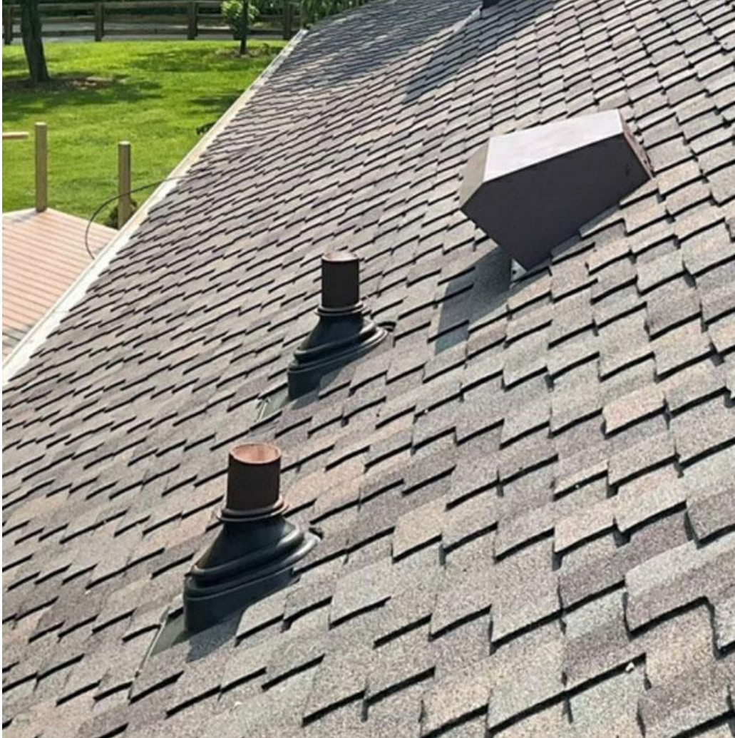
Newman Roofing, LLC installation showing The Ultimate Pipe Flashing®
