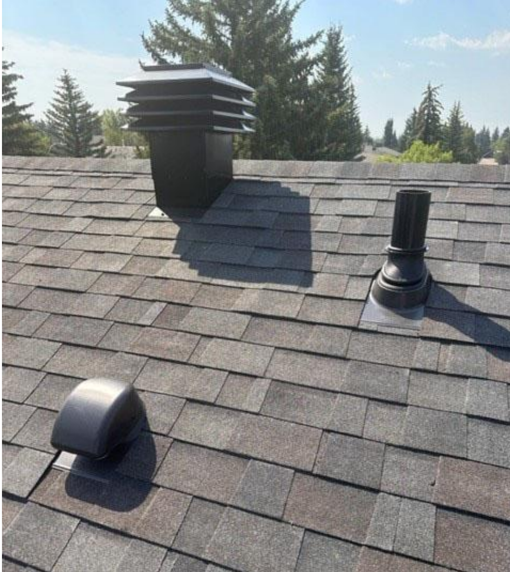
Bricor Roofing Ltd. installations of the Ultimate Pipe Flashing® and the Ultimate Bath/Dryer Vent
