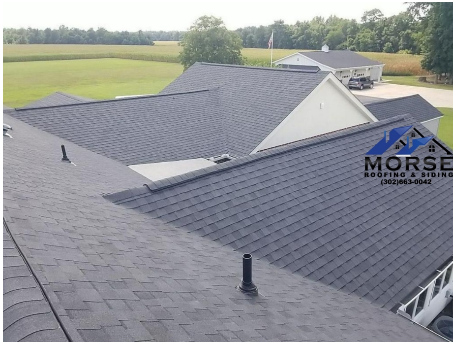
Morse Roofing & Siding
