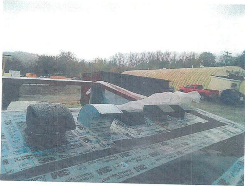
TOP OF DECKING
